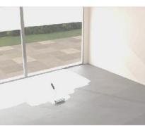
Prime the floor with acrylic based primer Leave to dry, typically 1 to 2 hours dependent of air temperature. Avoid excess foot traffic on primed surface.
