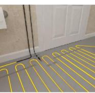
Now start installing the floor heating mat from the thermostat position. Roll out and secure the mat to the floor. The heating mat has a sticky mesh, simply press this down onto the floor and it will hold in place. If you need to turn the mat 90 degrees upside down you can use the double sided adhesive strips to hold the mat in place. A small amount of additional cloth tape is provided to ensure the mat is flat to the floor in places where it is uneven.
