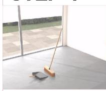
Ensure the sub floor is solid, suitable for tiling and free of dust and debris. Timber floorboards must be covered with a suitable thickness marine ply or suitable tile backer boards (PLEASE CONTACT FOR ADVICE IF YOU ARE UNSURE)
